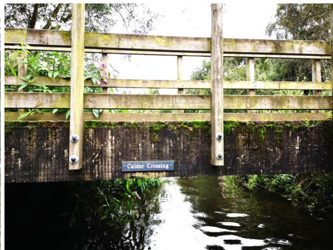
FOOTBRIDGE - SIDE FACING DOWNSTREAM.
