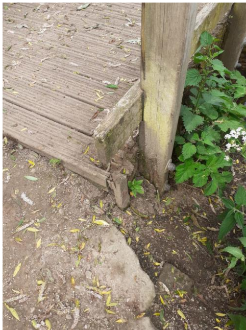
VIEWPOINT A – WET ROT AT LOW-LEVEL TO FRONT RIGHT-HAND AREA TO TIMBER DECKING & ADJACENT POST. (SEE DIAGRAM POINT 1).
