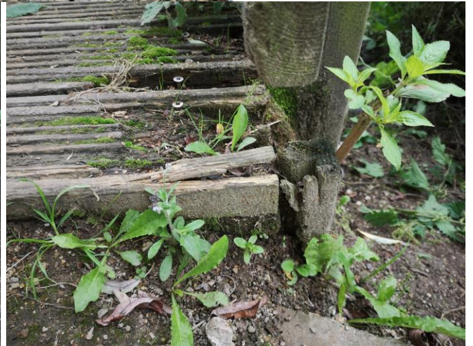
VIEWPOINT A – WET ROT AT LOW-LEVEL TO FRONT RIGHT-HAND AREA TO TIMBER DECKING & ADJACENT TIMBER POST. (SEE DIAGRAM POINT 1) GROUND FALLEN AWAY ADJACENT TO BRIDGE ABUTMENT.
