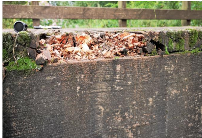
VIEWPOINT B – WET ROT AT LOW-LEVEL TO FRONT RIGHT-HAND CORNER POST. (SEE DIAGRAM POINT 2) GROUND FALLEN AWAY ADJACENT TO BRIDGE ABUTMENT.
