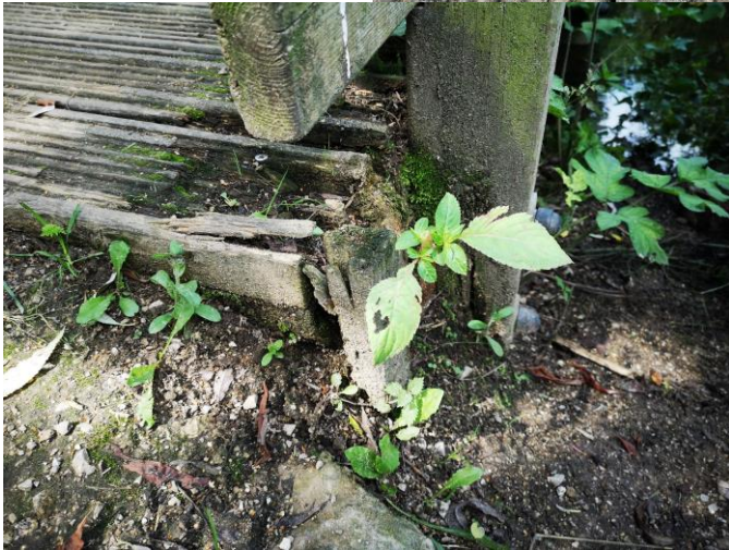
VIEWPOINT A – WET ROT AT LOW-LEVEL TO FRONT RIGHT-HAND AREA TO TIMBER DECKING & ADJACENT TIMBER POST. (SEE DIAGRAM POINT 1) GROUND FALLEN AWAY ADJACENT TO BRIDGE ABUTMENT.
