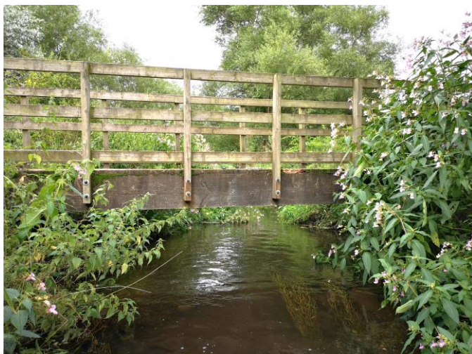
FOOTBRIDGE - SIDE FACING UPSTREAM.
