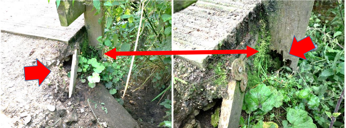
VIEWPOINT B – WET ROT AT LOW-LEVEL TO FRONT RIGHT-HAND CORNER POST. (SEE DIAGRAM POINT 2) GROUND FALLEN AWAY ADJACENT TO BRIDGE ABUTMENT.
