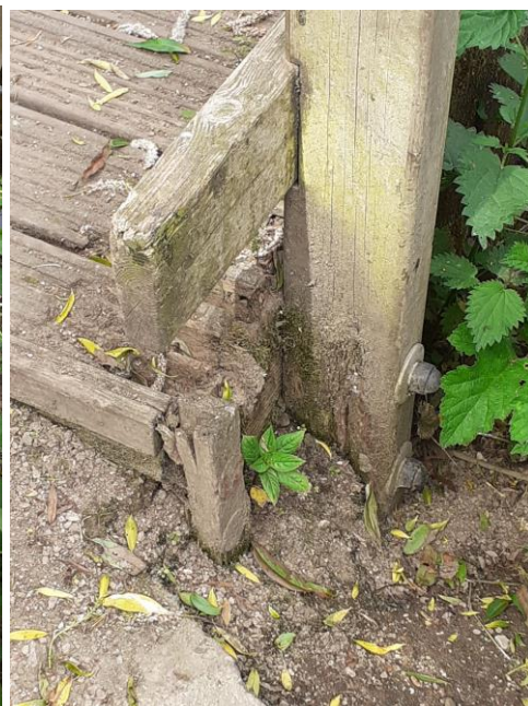
VIEWPOINT A – WET ROT AT LOW-LEVEL TO FRONT RIGHT-HAND AREA TO TIMBER DECKING & ADJACENT POST. (SEE DIAGRAM POINT 1).
